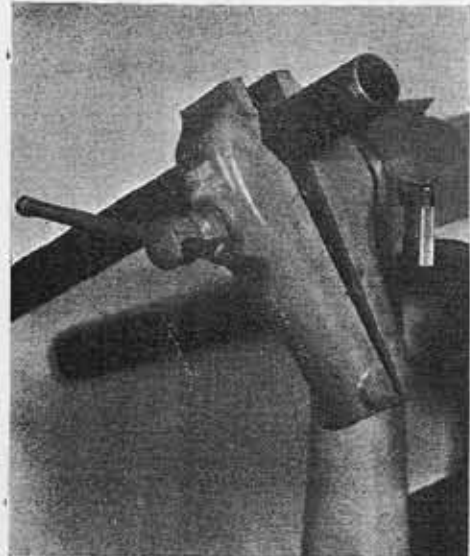
POSITIONING PIPE AND WELDERS VISE
